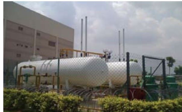
Pemasangan Gas Petroleum Cecair (LPG)
